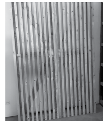
CLADDING: timber battens
